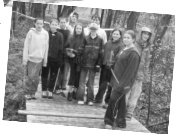
Sixth graders from Lyman Moore work through the rain to build a bridge extending the Lyseth/Moore School Trail to Pine Grove Park.
